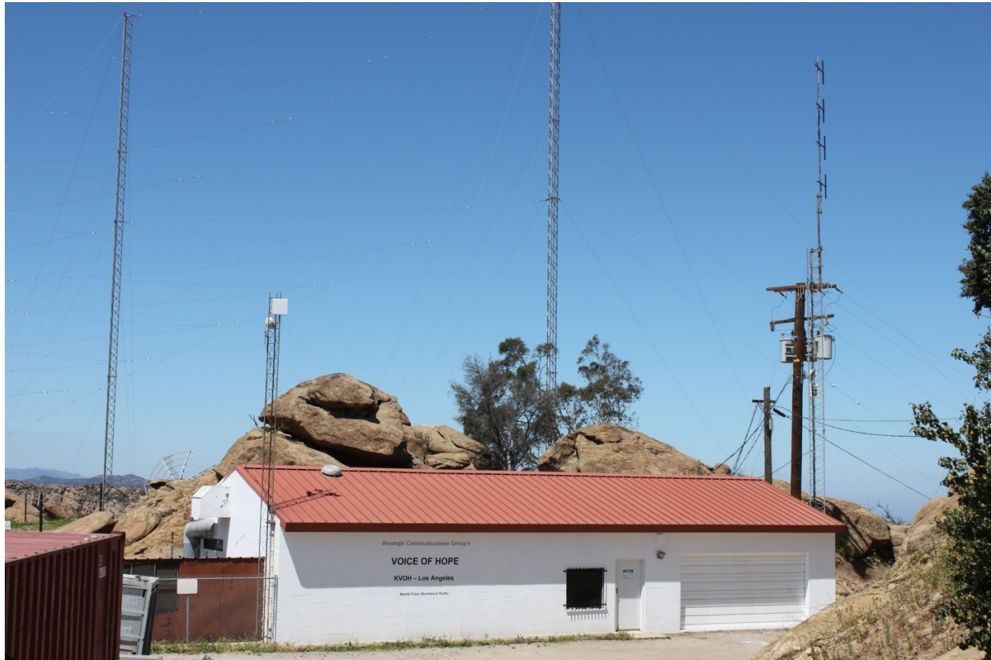
Transmitter Hall and TCI Log Periodic Antenna
